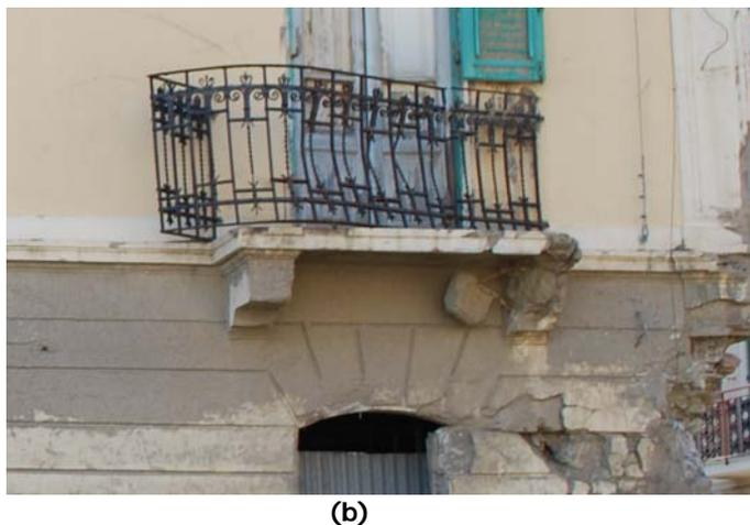
**Figure 20.** a) Comparison between analysis result and the observed damage for the Eastern wall, b) Deformation of the balcony in the eastern side of building.
